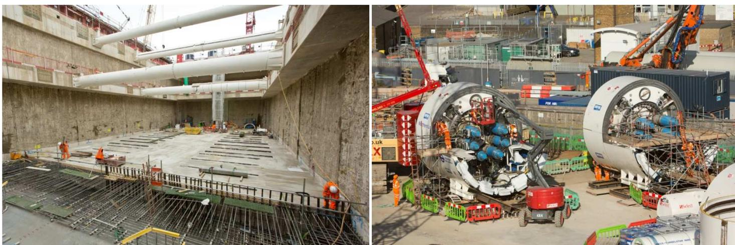
Between the crossover and station box, a temporary bridge has been constructed in line with the traffic site entrance to help facilitate site logistics over the months ahead. The approach ramps to this bridge have been constructed. Further west in the station box, the 100<sup>TH</sup> diaphragm wall panel has been constructed and the bored piles are ongoing.
