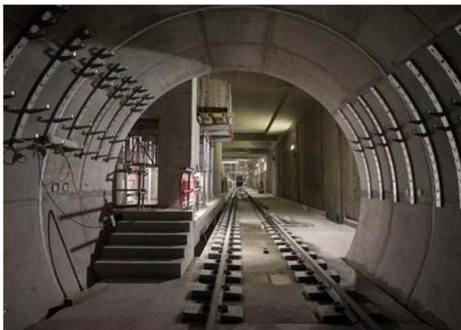
Fig 2. View of the platform from the overrun tunnel showing fit out works
