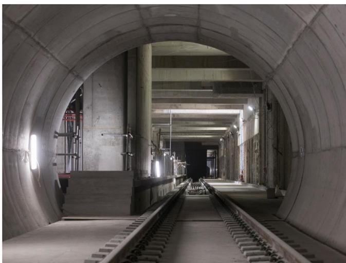
Fig. 1 Platform and track installation at the NLE Battersea site
