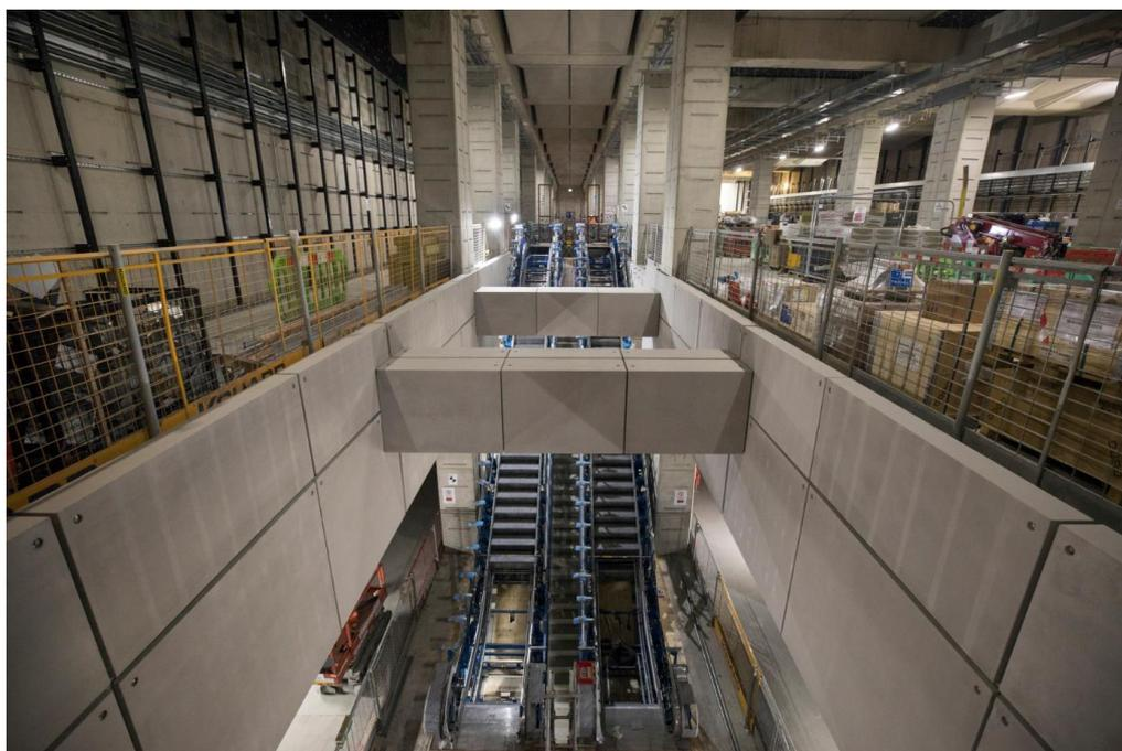
Fig 1. First bank of escalators installed
