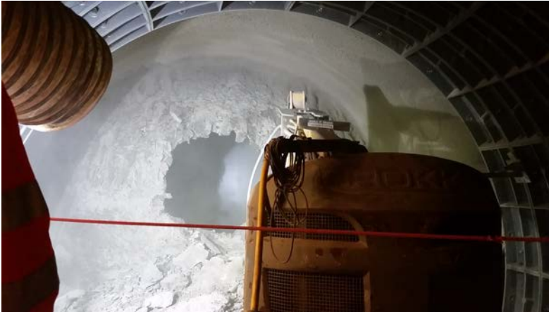
Tunnelling breakthrough at Bond Street station upgrade
