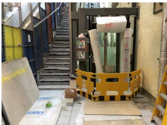
Lift works in progress at Greenford station
