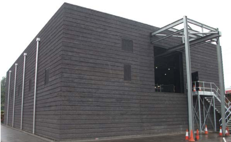
New West Ham high voltage substation
