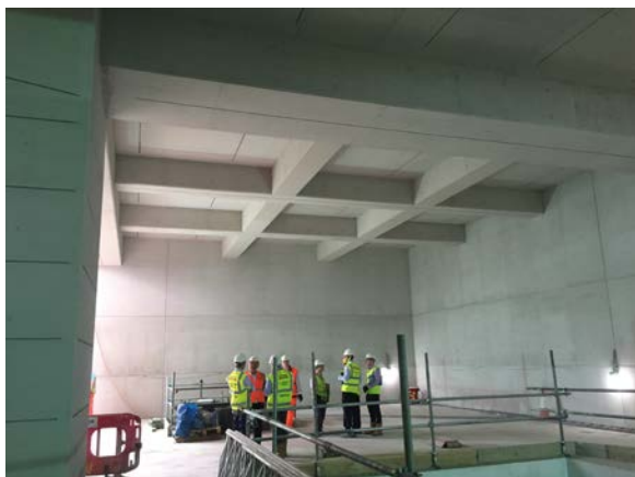
Station box – mezzanine level
