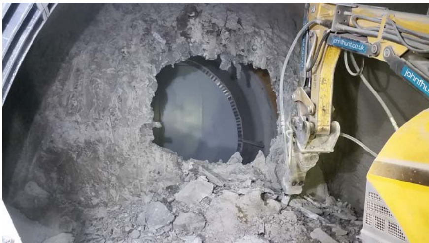
Tunnelling breakthrough at Bond Street station upgrade
