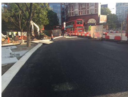
New widened carriageway at London Road junction
