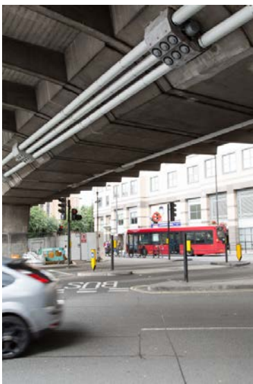
Expansion joint installation at Hammersmith flyover
