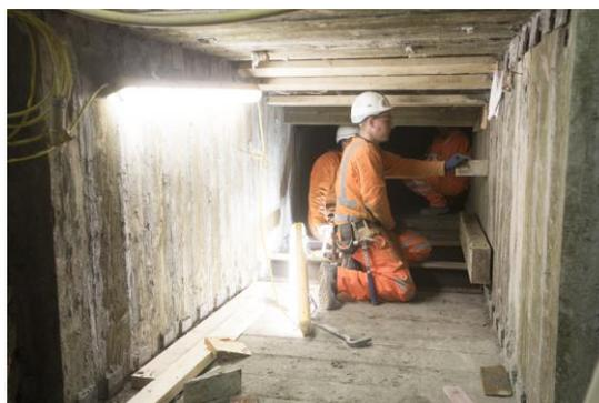
*Above – Image of a mechanical clay spade used for excavating the 6.5m tunnel and works on the tunnel support.*
