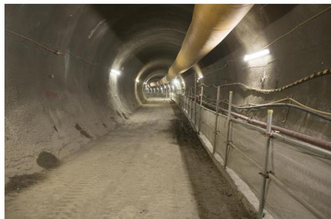
*Above – images of the tunnel support works and the Sprayed Concrete Lining tunnels*
