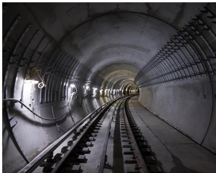
Fig. 2 Completed conductor rail installation
