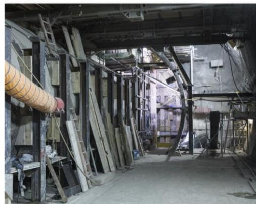
*Above – image of the installation of the SGI rings and the tunnel support works.*
