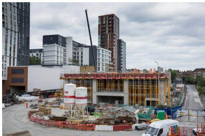
Fig.2 Final concrete pour to complete the roof of the western superstructure
