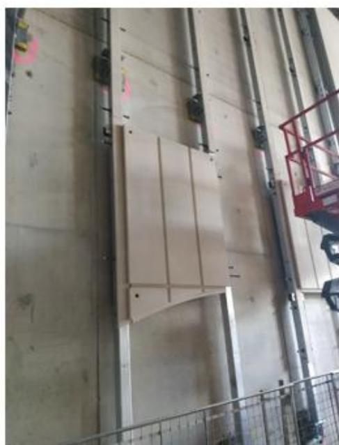
Fig.3 Cladding works underway at ticket hall level
