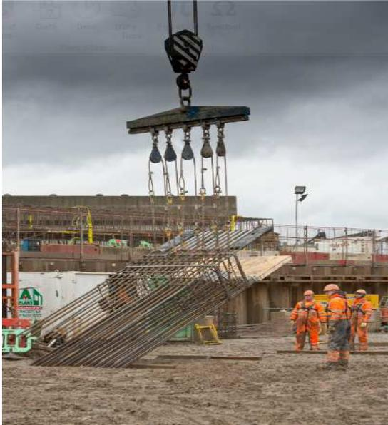
The Diaphragm wall cage being lifted to position for installation
