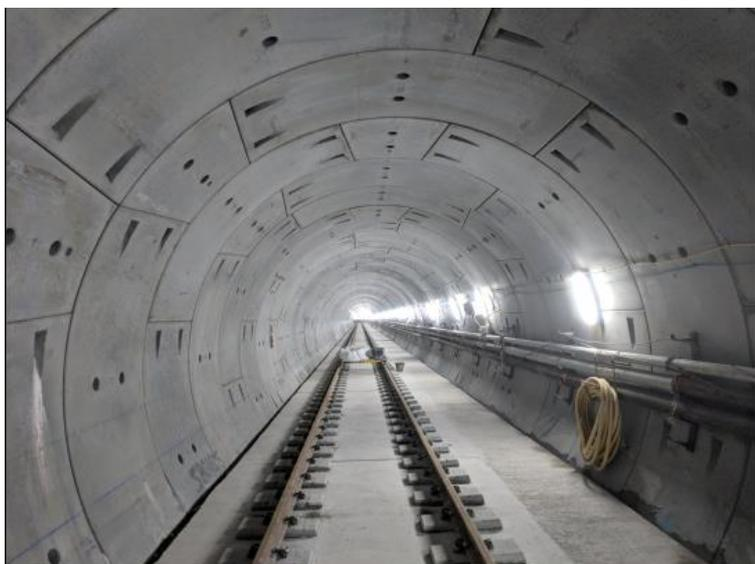
Fig. 1 Track installation plus Cess walkway
