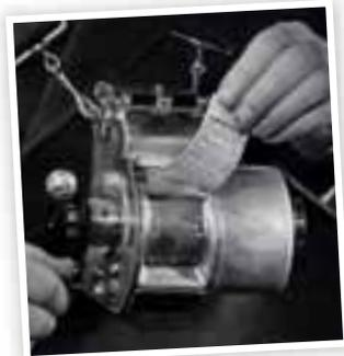
The machine was named after its inventor, the late George Gibson, a one-time superintendent of Stockwell punch works. It was a simple machine, built for London Transport requirements, with a range of 14 possible fares – which was expanded at a later date. Various dials recorded the numbers of each denomination
