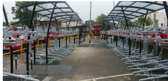
Figure 7: Example of two-tier racks installed in a station car park
