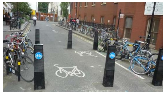
Figure 4: Cycle parking installed as part of a modal-filter
