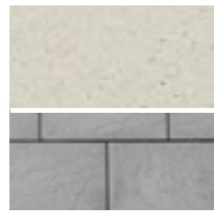
Floor tiles/pavers Terrazzo (int) Concrete flagstones (ext)
