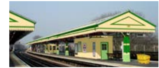
Ravenscourt Park Painted timber platform canopies
