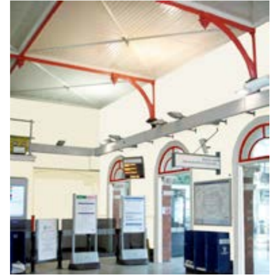
Plaistow ticket hall Painted ironwork, glazing bars and timber plank soffit
