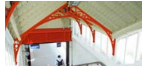
Roof ironwork (Plaistow)
