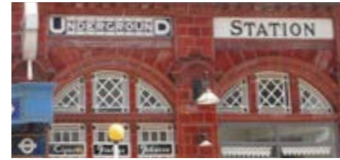
Glazed oxblood faience, terracotta facade with arch windows, exterior wall mounted light and original underground sign
