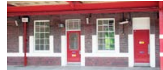
Becontree Fletton brick with painted timber doors
