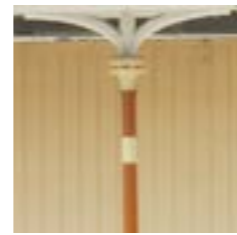
Cast iron Canopy supports (plat)
