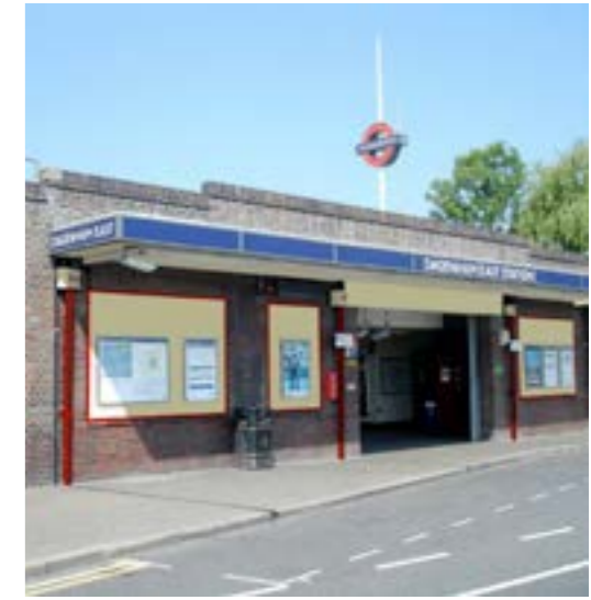
Dagenham East Fletton brick façade with blue canopy
