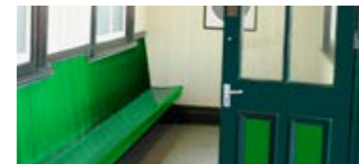
West Finchley Waiting room interior showing cream and green painted timber walls
