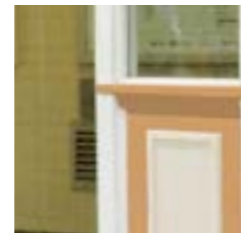
Timber Painted panels/ Dados/window frames
