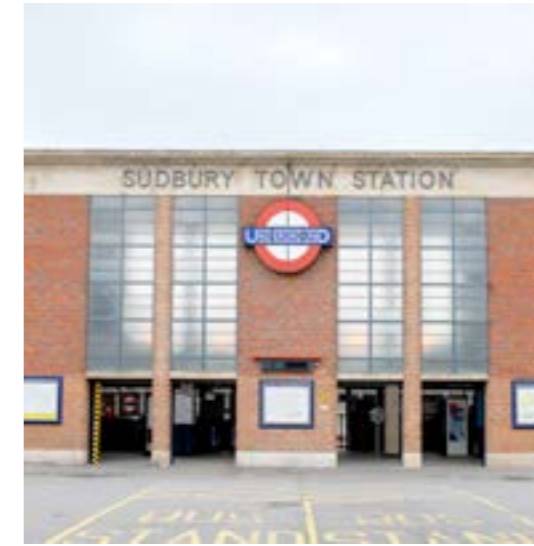
Sudbury Town exterior
