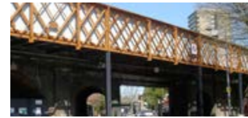
Lattice bridge details (Latimer Road)
