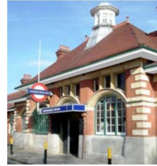
Barkingside Red brick with stone corner details and clay roof tiles
