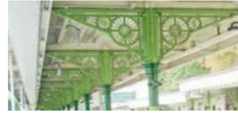
Decorative brackets (Snaresbrook)
