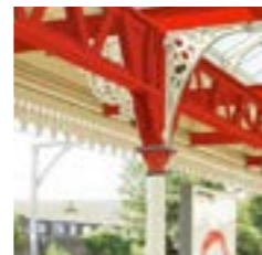
Cast iron Canopy supports (plat)
