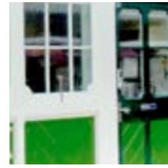
Timber Painted panels/ Dados/window frames
