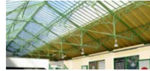
Roof trusses and framework (Ealing Broadway)
