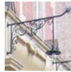
External wall mounted light (Queensway)
