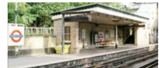
Woodside Park platform and platform building London stock brick platform with cast iron and timber canopy
