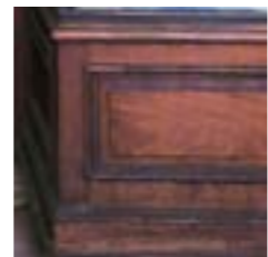
Varnished timber (Clapham South)
