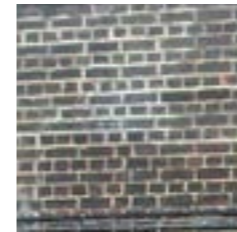
Brick construction Flemish bond (station specific)
