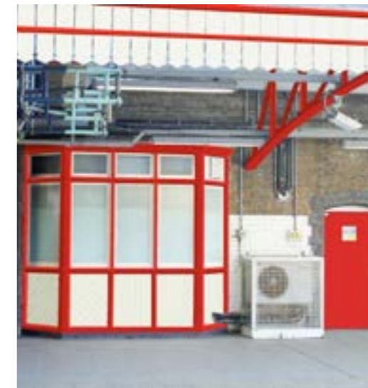
Bow Road platforms Painted ironwork and timber canopy
