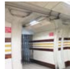
Painted plaster portal frame (Regent's Park)
