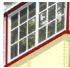
Timber Painted sills / window frames
