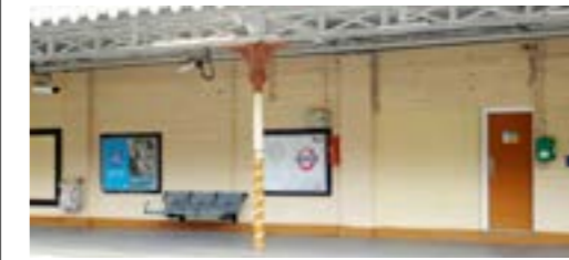
Westbourne Park Painted columns and platform walls in station colour scheme
