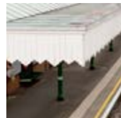
Timber Painted pailing fences/ valance (plat)
