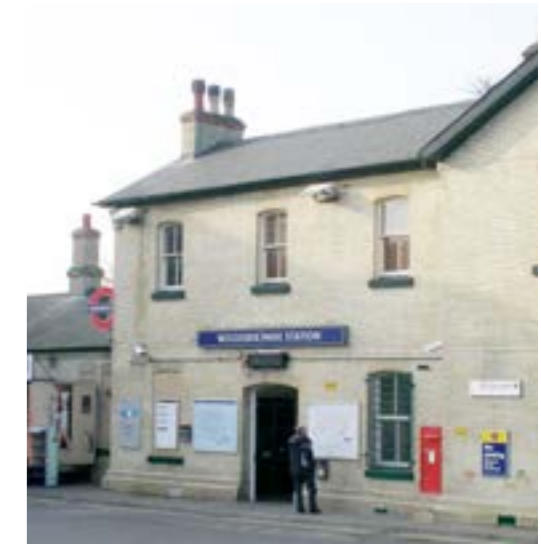
Woodside Park Stock brick station exterior with painted white window frames and dark brunswick green sills and doors. Slate pitched roof
