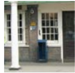
Timber Painted sills/ window frames (Croxley)
