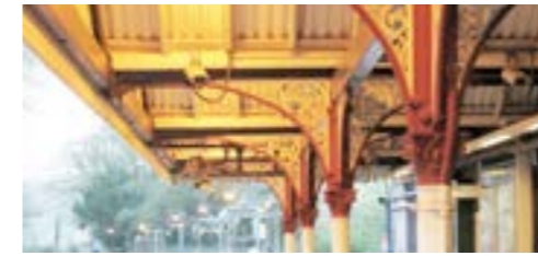
Decorative brackets (Chesham)
