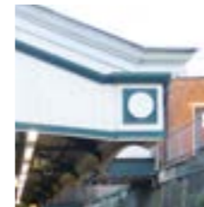
Platform canopy detail (Colindale)
