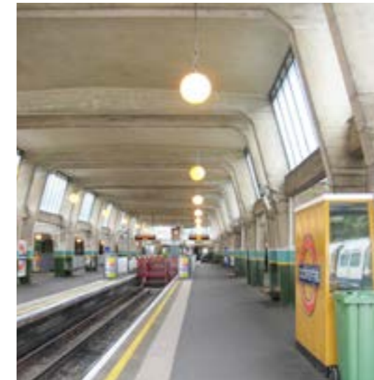
Cockfosters train shed interior
