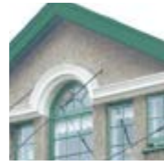
Timber Painted cills/window frames/ external architrave
