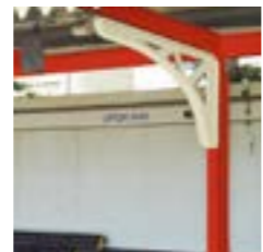
Cast iron Canopy supports (plat)
