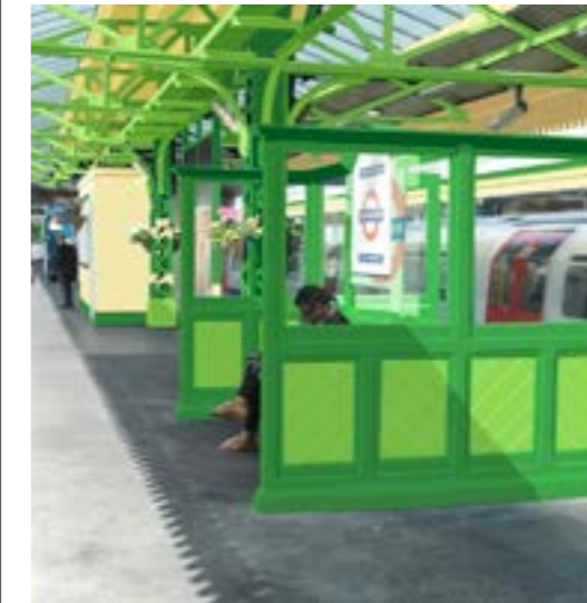
Turnham Green painted timber platform screens.
