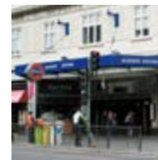
Entrance canopy (Aldgate)
