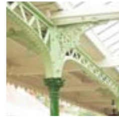
Cast iron Canopy supports (plat)
