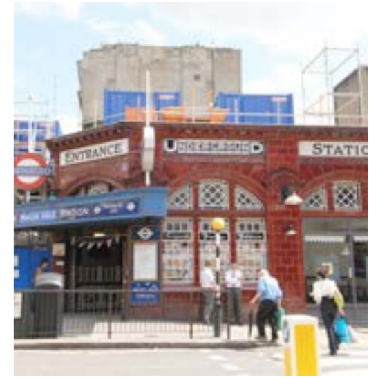
Maida Vale station exterior
