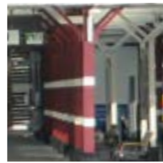
Steel Canopy supports (plat) (Watford)
