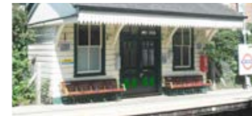
West Finchley Timber clad platform building with timber and canopy and slate roof
