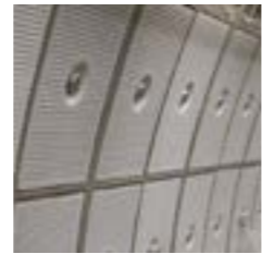
Tunnel forming rings and stove enamelled plates (Westminster)
