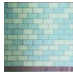
Tiled panels Willesden Green (tiles int)
