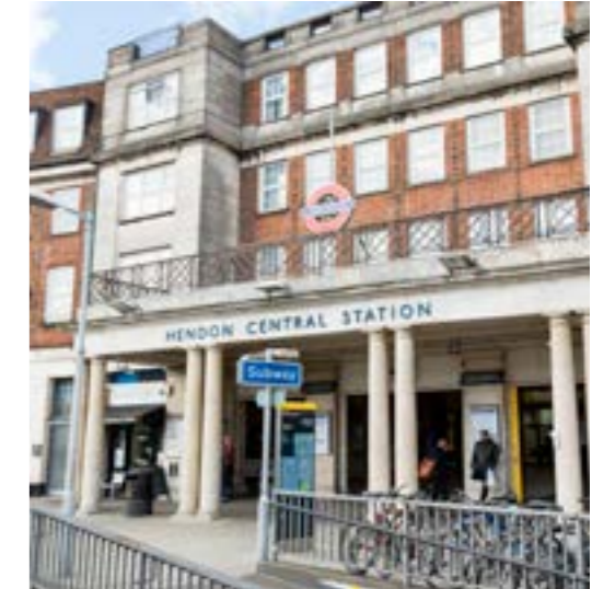
Hendon Central exterior
