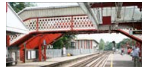
Lattice Bridge (Amersham)
