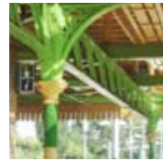
Cast iron Canopy supports (plat)
