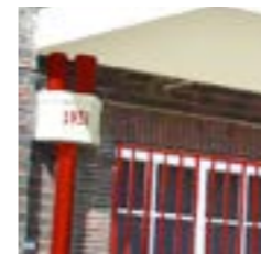
Rainwater hopper (Hornchurch)
