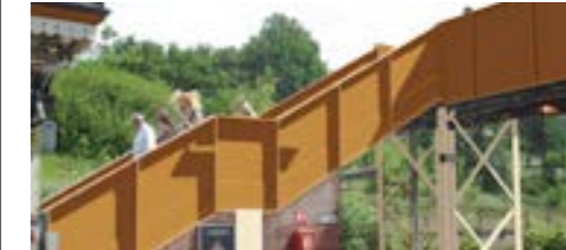
North Acton Painted metalwork footbridge in station colours
