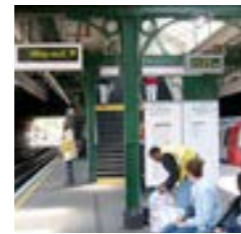
Cast iron Canopy supports (plat) (Willesden Green)
