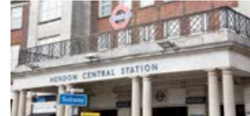
Neo-Georgian columns, bronze balcony hand rails and lettering (Hendon Central)
