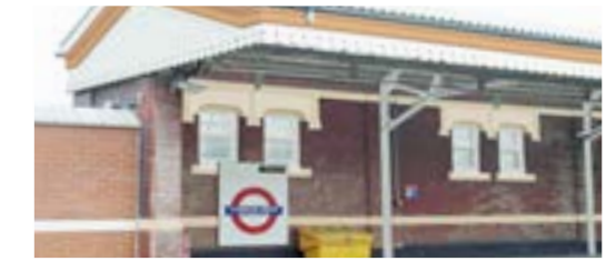
Ladbroke Grove Brick platform walls and painted timber canopy detail
