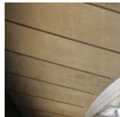
Precast concrete panelling
