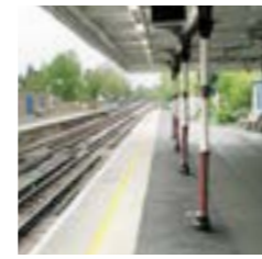
Cast iron Canopy supports (plat)
