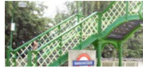
Lattice bridge details (Barkingside)
