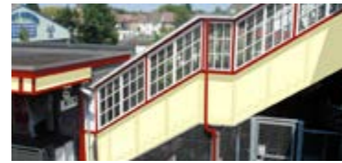
Riveted steel paneled fully enclosed stairs (Dagenham East)
