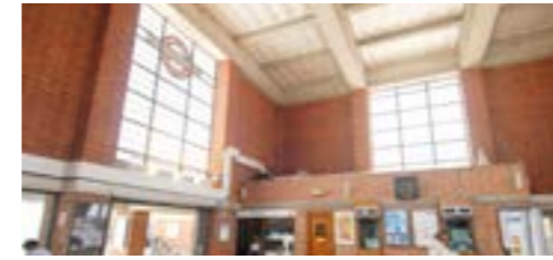
Structure expressed interior and white painted ceiling (Sudbury Hill)
