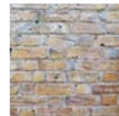
Brick construction Flemish bond (Chalfont & Latimer)
