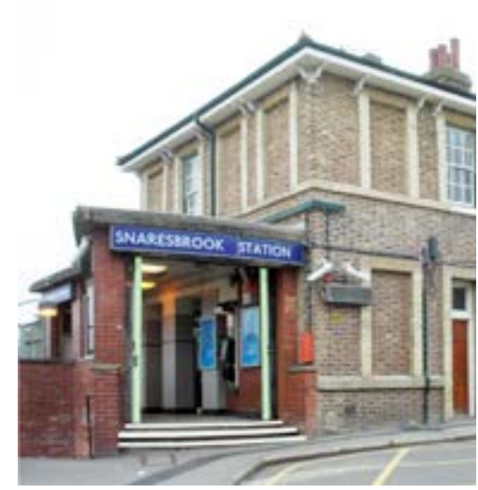
Snaresbrook London stock brick façade with buff brick window and door surrounds
