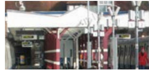
Inverted pitched platform canopy (Watford)
