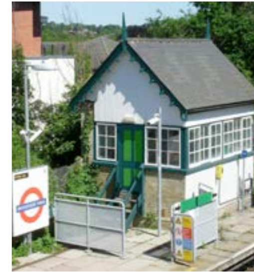
Woodside Park Painted timber and London stock brick ancillary building displaying the details and approach to colour composition
