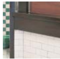
Varnished timber (Warwick Avenue; route ways)
