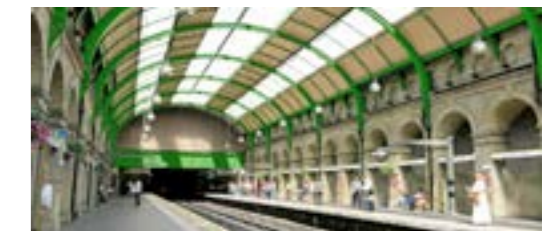
Notting Hill Gate Cast iron painted arch and glazed roof
