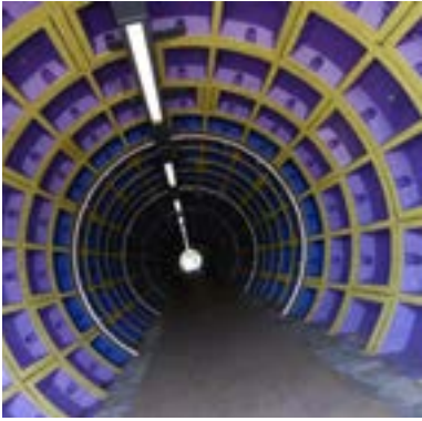
Circular tunnel forming rings
