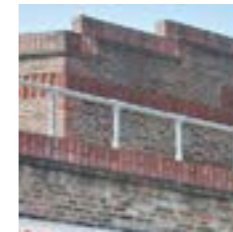
Façade brickwork (Upminster Bridge)
