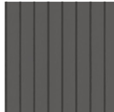
Painted vertical tongue and groove panelling
