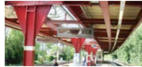
Structural brackets (Upminster Bridge)
