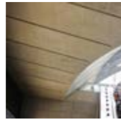
Precast and in-situ exposed concrete (Canary Wharf)
