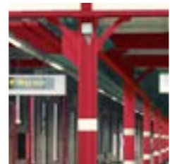
Steel Canopy supports (plat)
