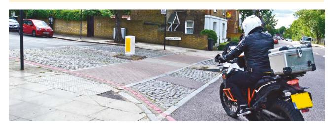
This entry ramp is set back from the main carriageway, so for a motorcyclist the road surface doesn't change until the manoeuvre is almost completed. However, towards the end of the manoeuvre, on the up ramp, there are potentially slippery granite setts which can cause problems especially when wet.
