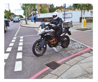
The braking area on the approach to the junction has a granite sett down ramp, which is poorly maintained and has substandard reinstatement where it has been repaired.
