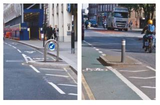
The build-out forms a strike hazard, with the steel hoop forming an unforgiving structure if hit by a motorcyclist.
