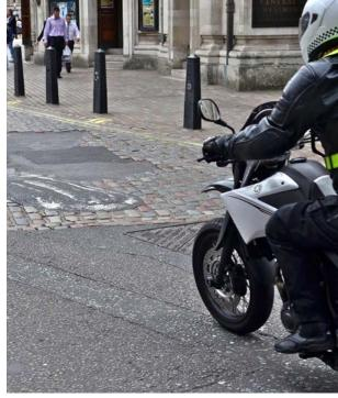
Here there are four different road surfaces within close proximity. Tarmac, inspection covers, worn thermoplastic on a raised oval of tarmac (with no warning) and cobbles. In an area with a high pedestrian flow and busy traffic lanes, this will cause stability problems for motorcyclists.
