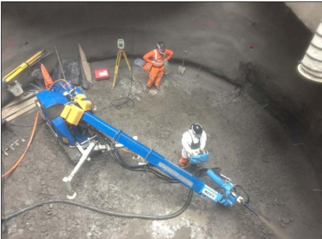
*Bond Street concrete lining spray of shaft 1*
