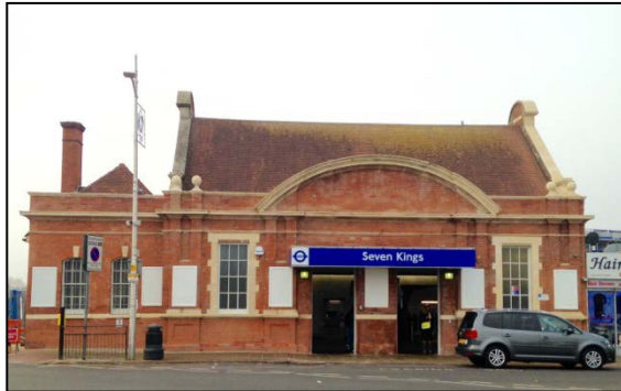
Seven Kings – External clean & repair
