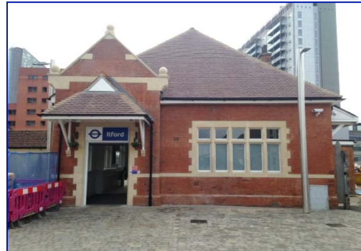
Ilford York Road – New station entrance
