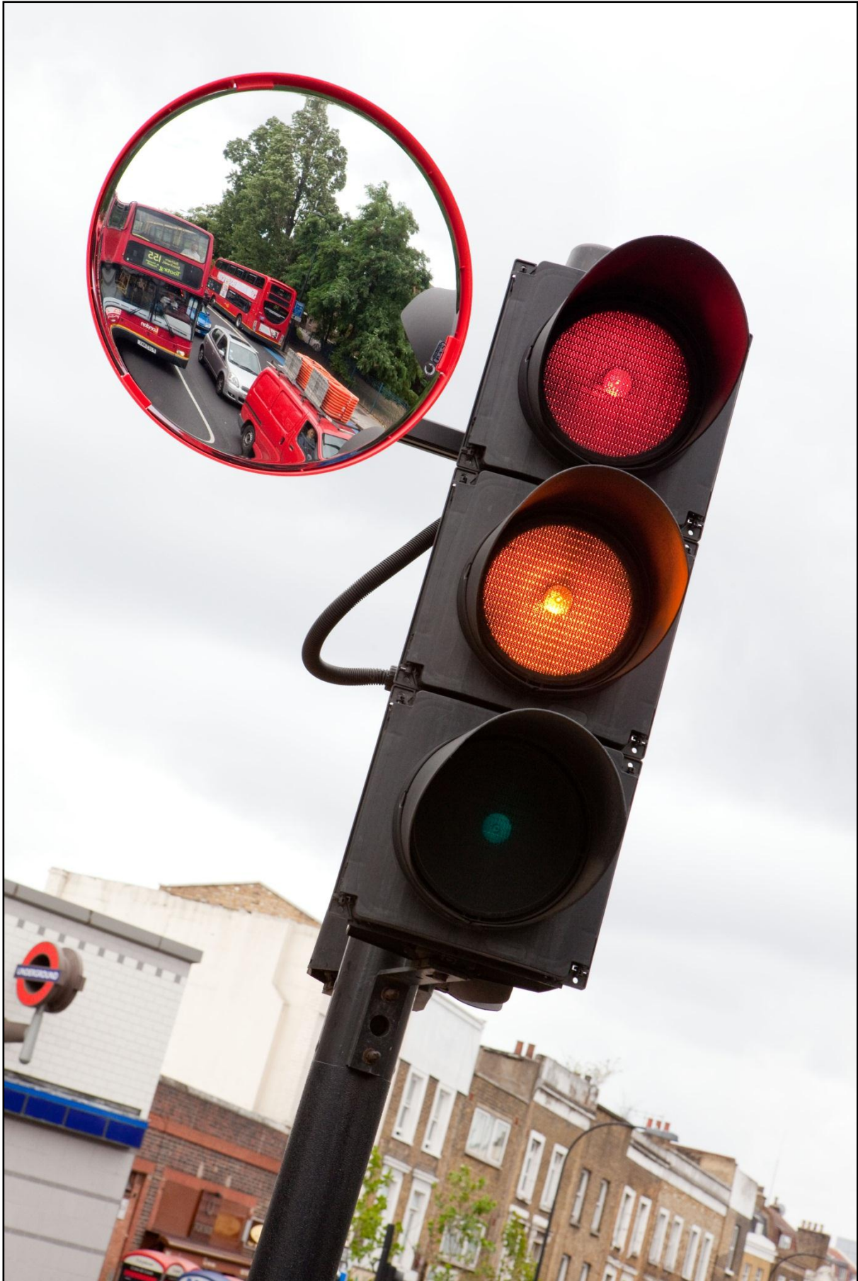
We will convert traffic signals to LED extra low voltage
