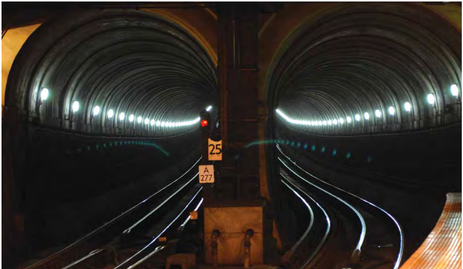
The Thames Tunnel, built by Sir Marc Brunel and his son Isambard between 1825 and 1843, will form part of the new £1 bn East London line and the London Overground network. More than 160 years after it was completed, it will carry London's latest fleet of 21st century commuter trains
