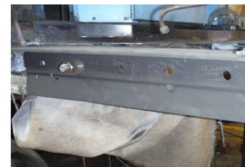
Sole bar repair
