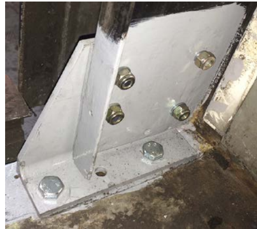
Internal door pillar repair
