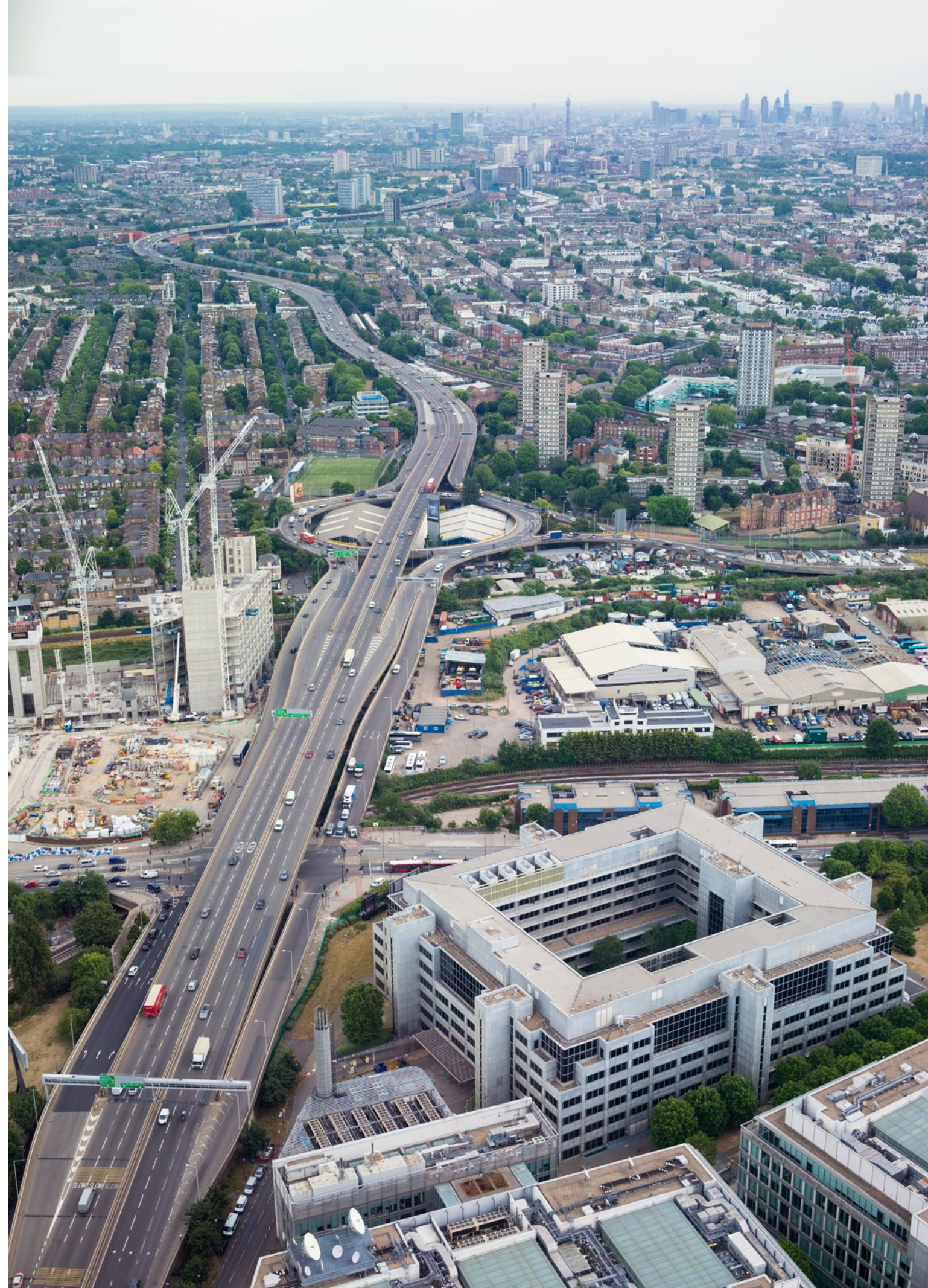
Repairs to the Westway keep this key highway safe and avoid disruption
