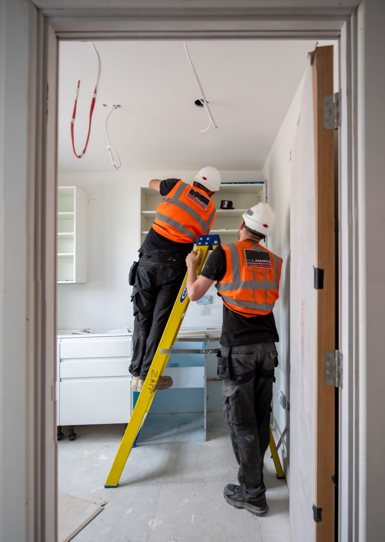
We are working to improve the thermal efficiency of our buildings
