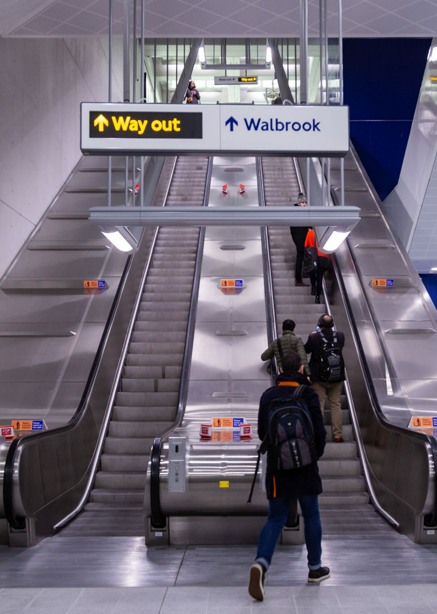
New escalators, moving walkways and lifts have improved access at Bank
