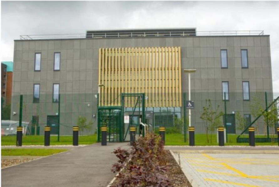
Romford Route Control Centre
