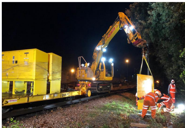
Figure 4: Traction Isolation Switches (TIS) being installed at Stonebridge Park Depot
