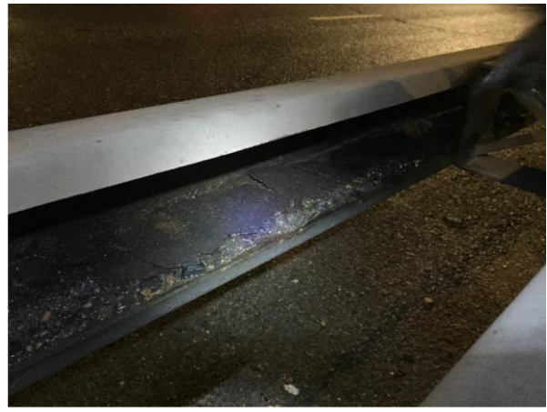
A40 Central Vehicle Restraint Barrier (VRS): Corrosion of supports and longitudinal restraints requiring speed restrictions
