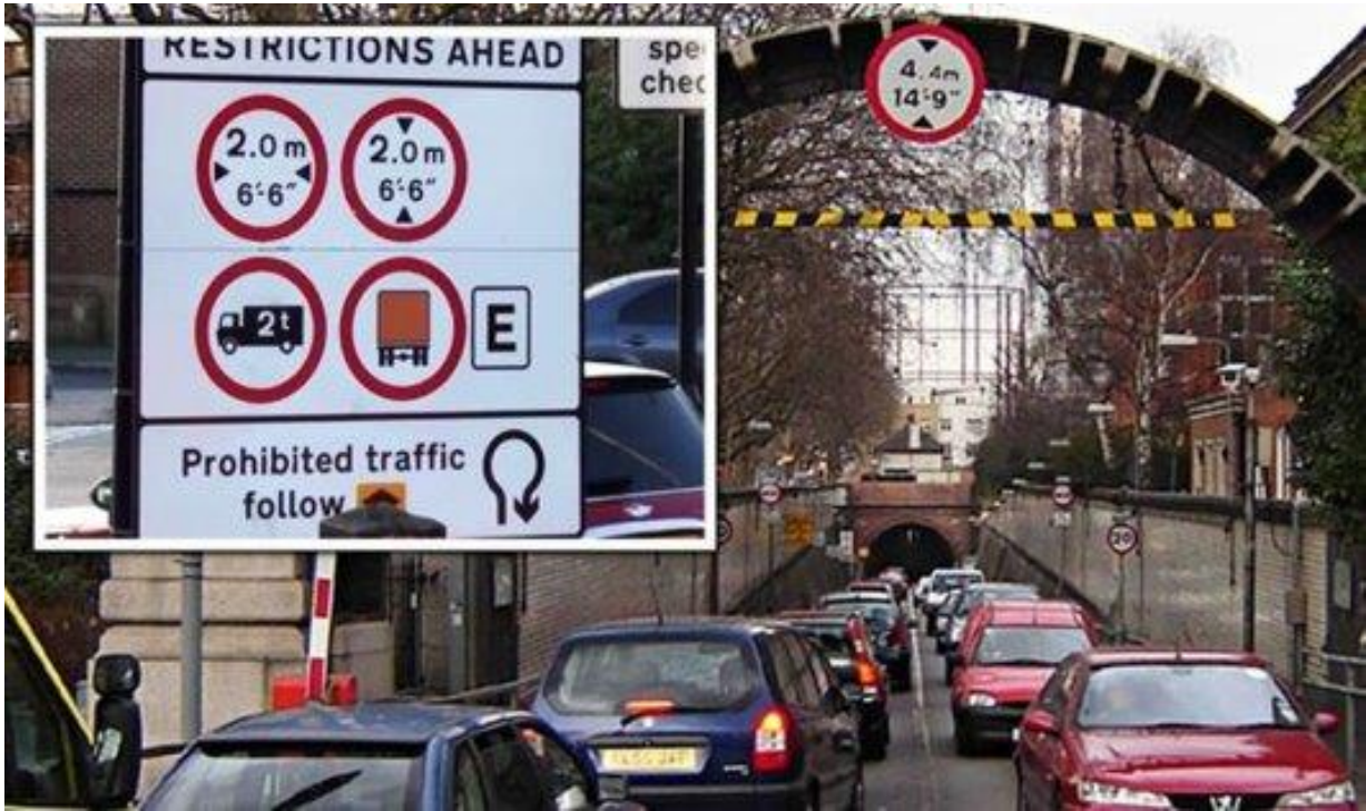
Rotherhithe Tunnel: restrictions already in-place due to aging
