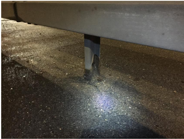
A40 Central Vehicle Restraint Barrier (VRS): Corrosion of supports and longitudinal restraints requiring speed restrictions
