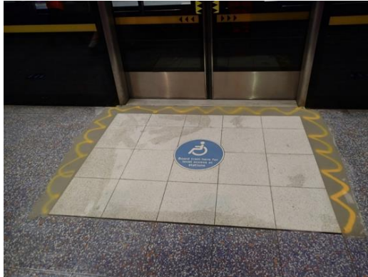
Figure 3: A Jubilee line platform being modified for level access
