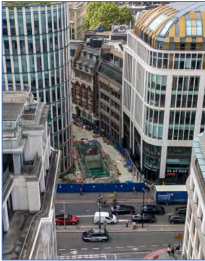
Figure 1: Arthur Street shaft (photo taken on May 2024, remains as is)
