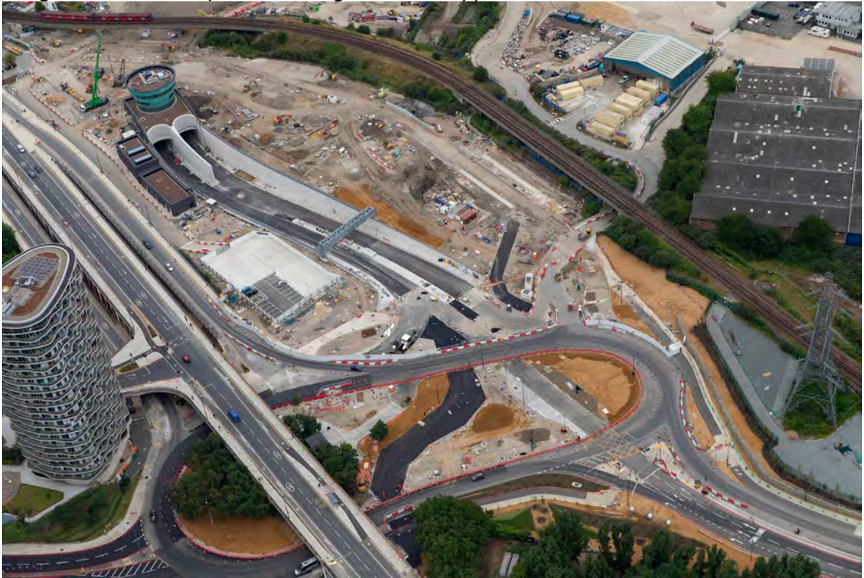
Image 7 - Silvertown portal building and north approach roads
