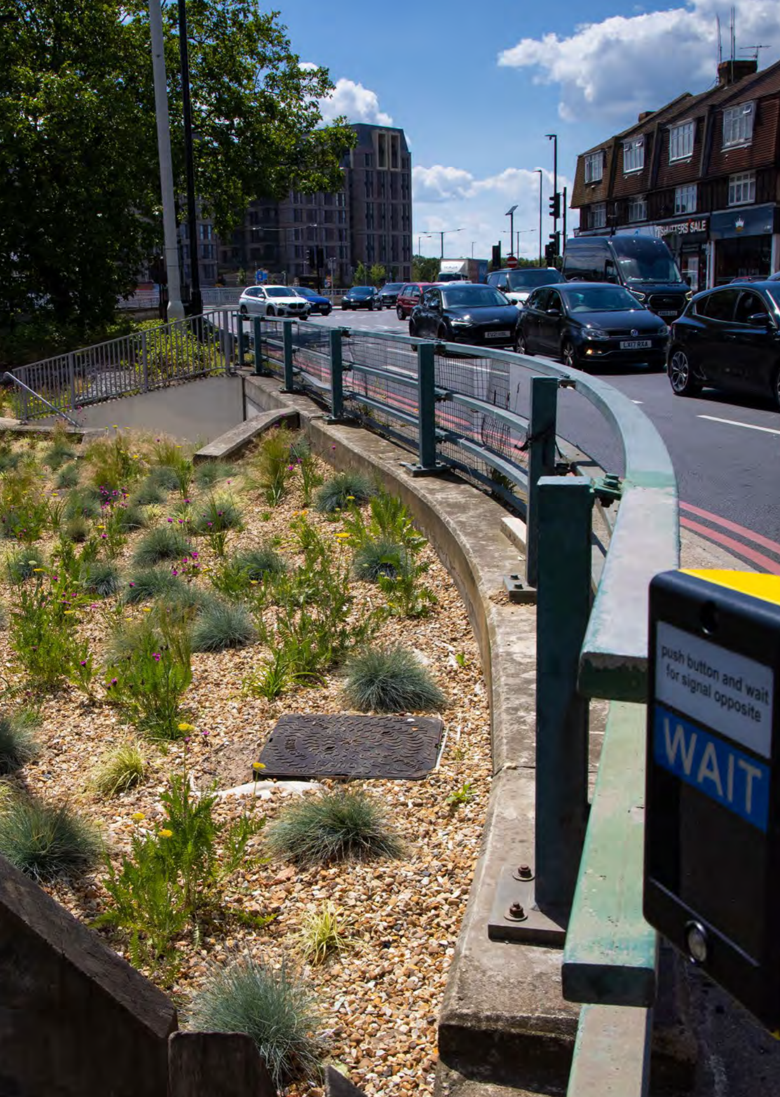
Sustainable drainage slows the rate of surface runoff to reduce flooding
