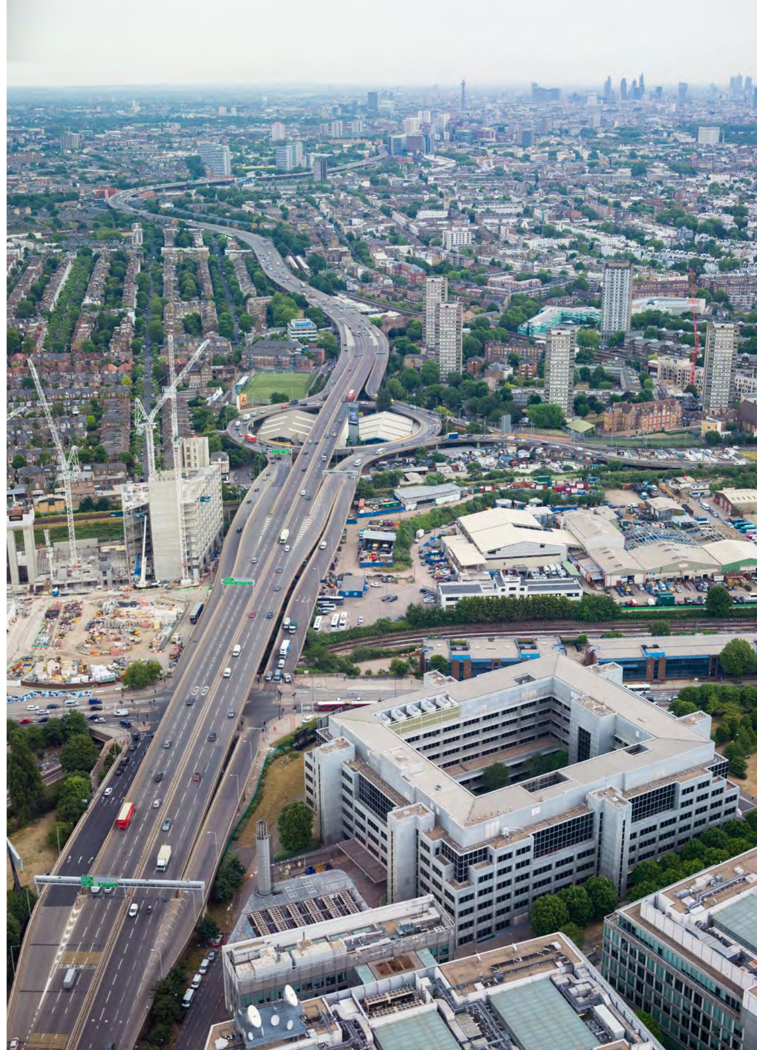
Repairs to the Westway keep this key highway safe and avoid disruption
