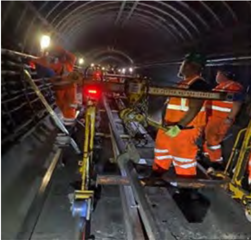
Figure 3: PLU Enabling Works progress:
