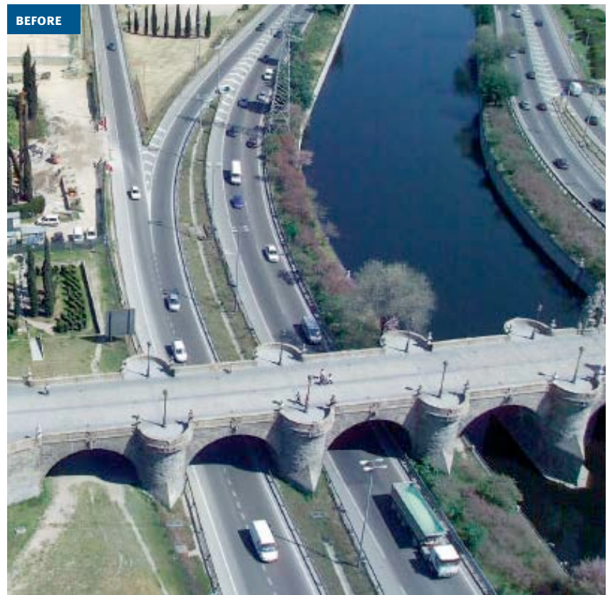
FIGURE A7.3 M-30 BEFORE TUNNELLING
