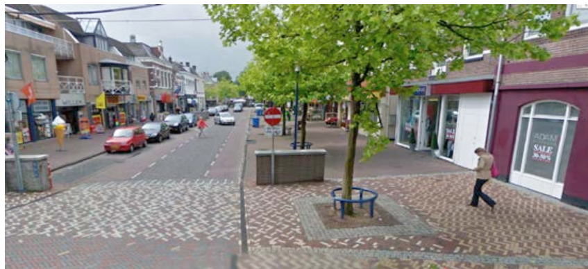
FIGURE A11.1 BICYCLE LANES IN BOTH DIRECTIONS IN THE CITY CENTRE, WITH ONLY ONE-WAY TRAFFIC LANE
