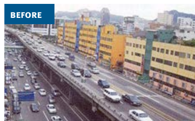
FIGURE A13.1 ELEVATED MOTORWAY COVERING THE STREAM
