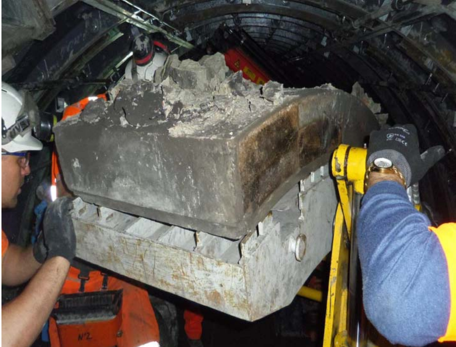
Ring segment being removed
