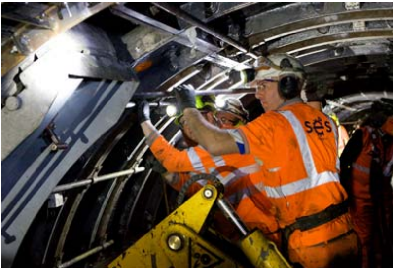
Baker Street to Bond Street tunnel relining
