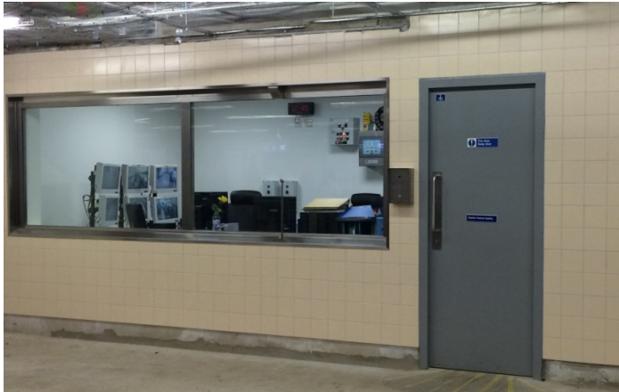
New station control room at Vauxhall
