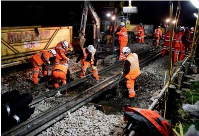
Track Partnership works
