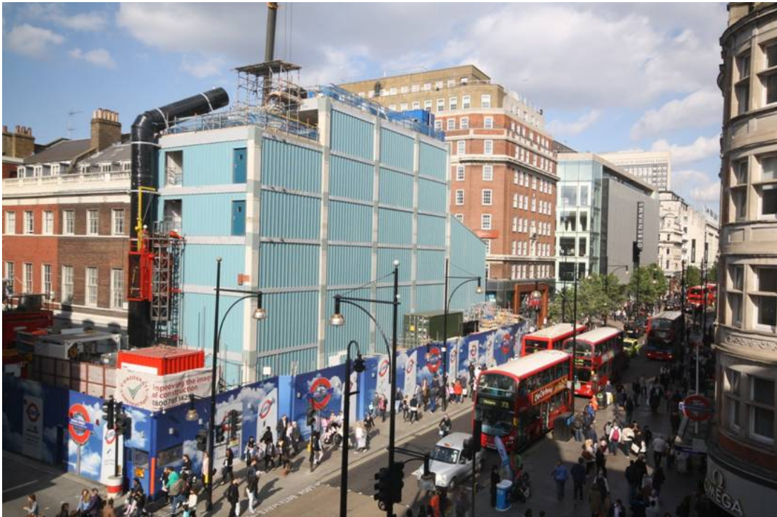
Progress on the over-site development at Bond Street
